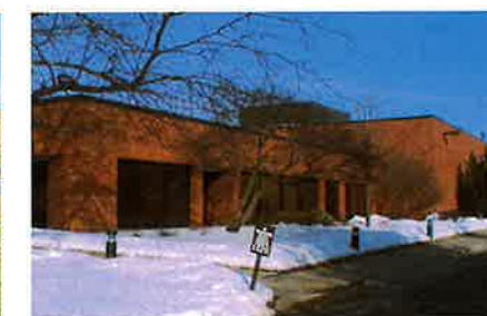
②-2 KANAFLEX CORPORATION of ILLINOIS (アメリカ) 875 Woodlands Pkwy Vernon Hills, IL 60061, USA
