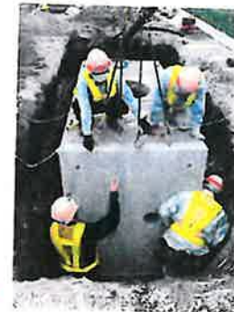
Kanacrete box culvert
